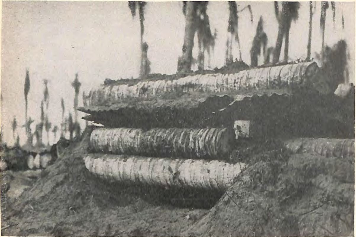
Figure 143. Exterior view of pillbox.
